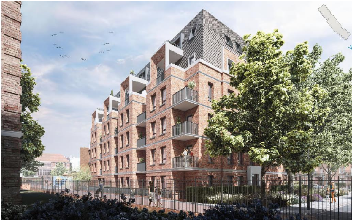
Image 7: View of Building B from Lisgar Terrace
